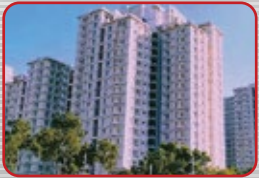
Rooppur Residential Village Pabna
