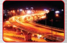
Mohakhali Flyover Dhaka
